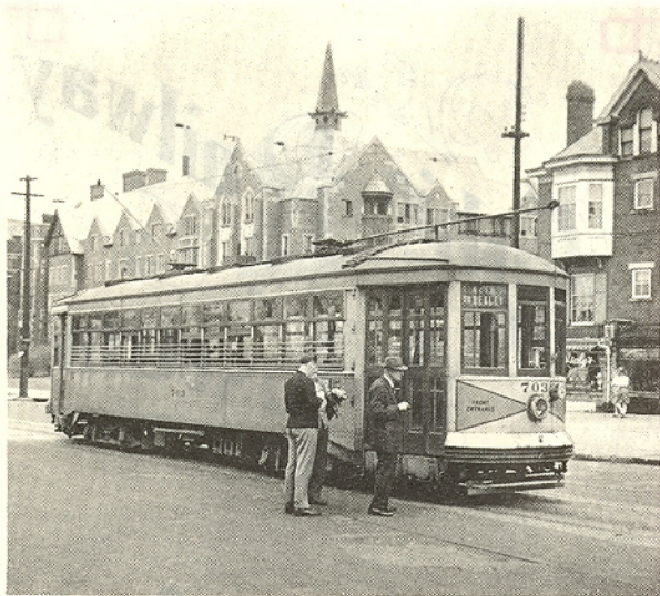
Columbus & Southern Ohio Electric Co. No. 703 at 11th and Neil Ave, 1948.
